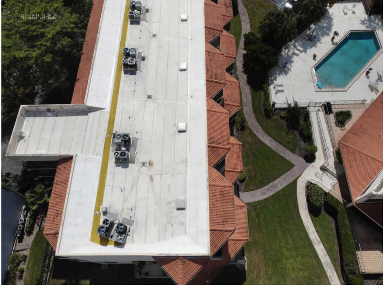
Drone Photo of Roofs captured 10/15/2021
