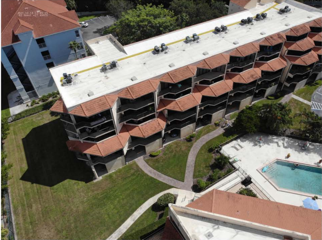
Drone Photo of Roofs captured 10/15/2021
