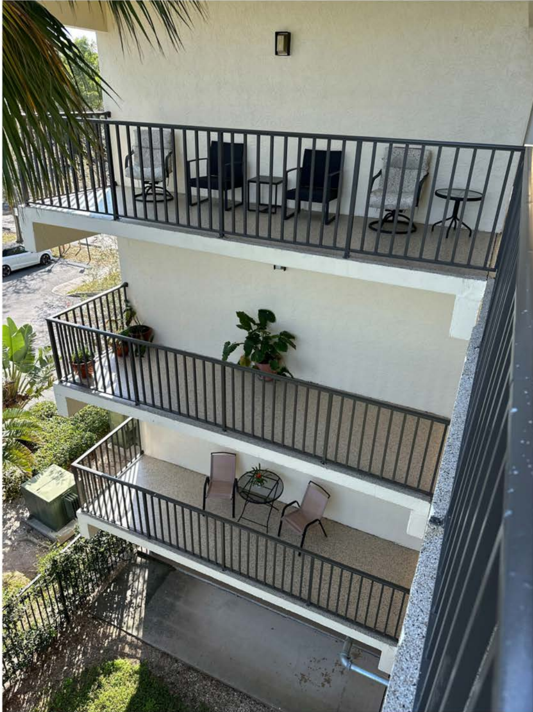
Exterior view of balconies captured on 2/24/2023
